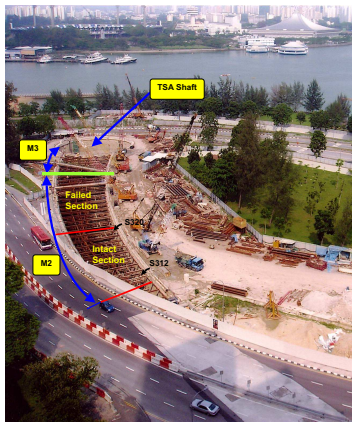
Overview of Affected Project Site Prior to Accident
