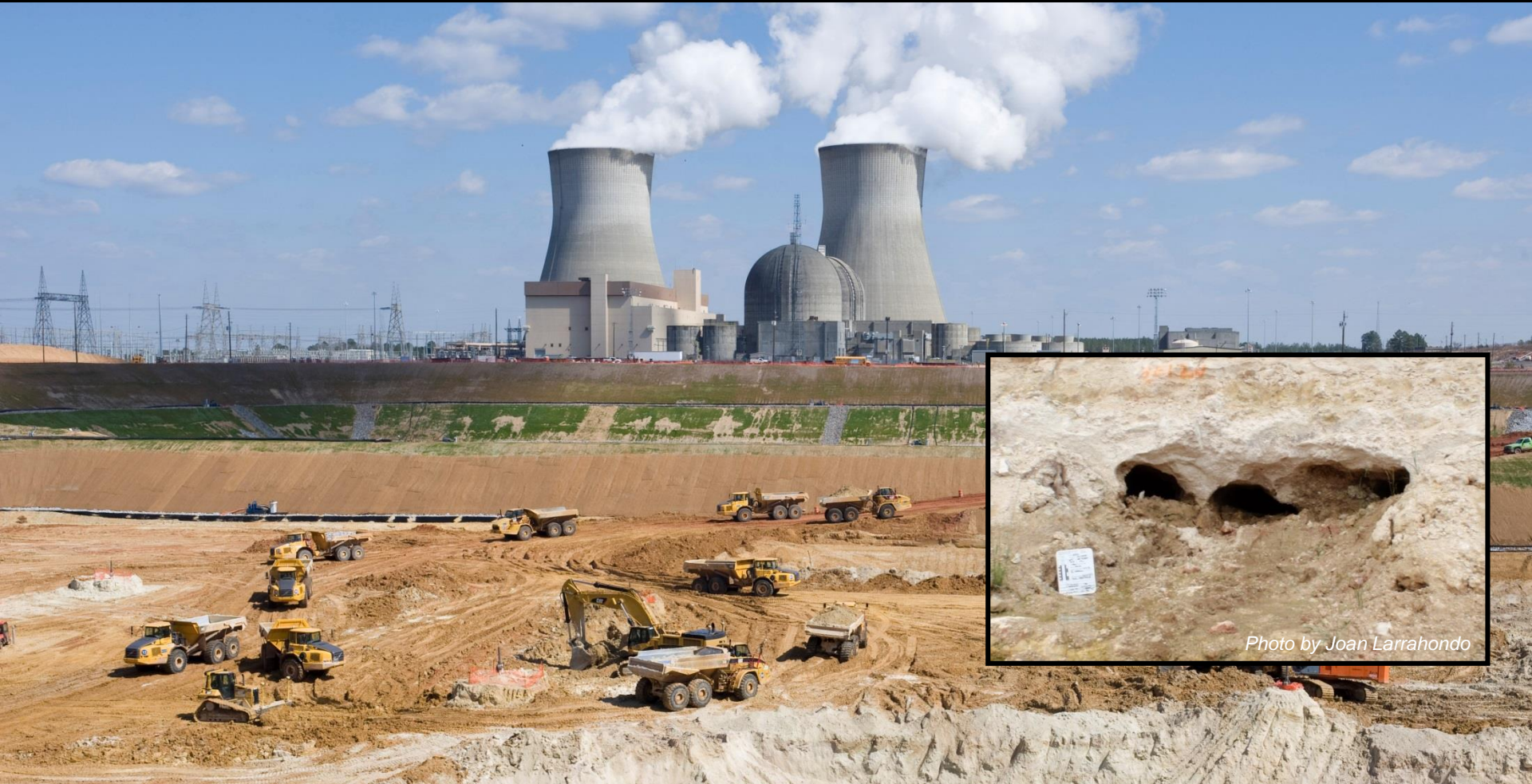
Plant Vogtle (GA) - Excavation Units 3 & 4 (Photo: Southern Company, 2010)
